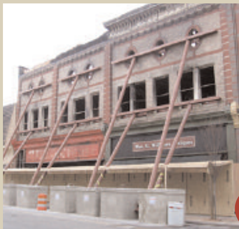
The stabilization system for the fire-damaged facade at 444-448 Race Street.
